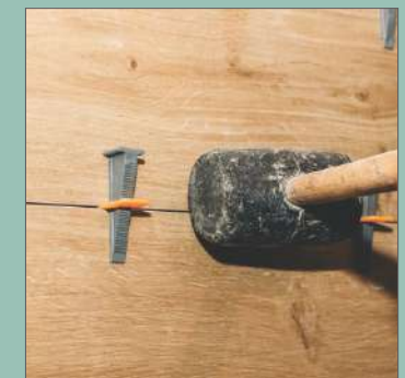
Remove Wedges Ones It Dry
