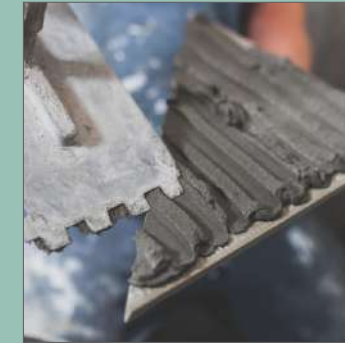
Cement Laying On Tile
