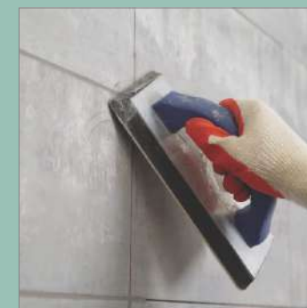
Joint Grouting
