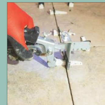
Levelling Wedges
